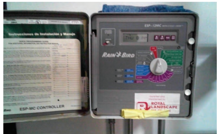
L7 - Existing irrigation controller
