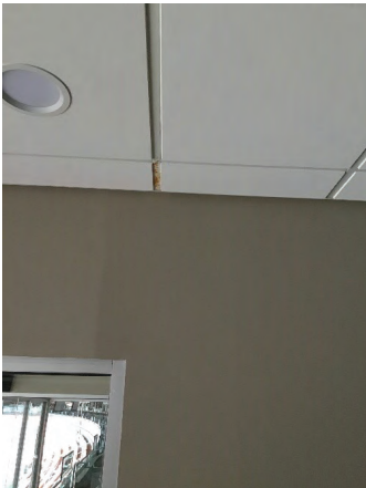
A8 - Water damage ceiling and grid
