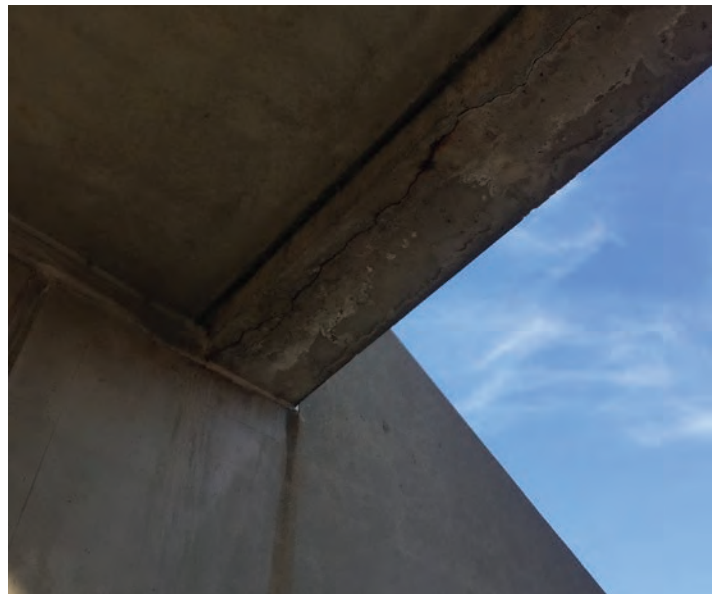
S2 - Typical Cracked Concrete
