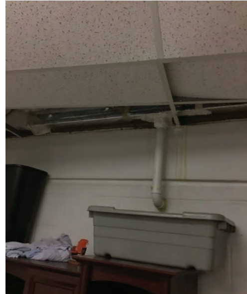
A13 - Water damage at finish ceiling
