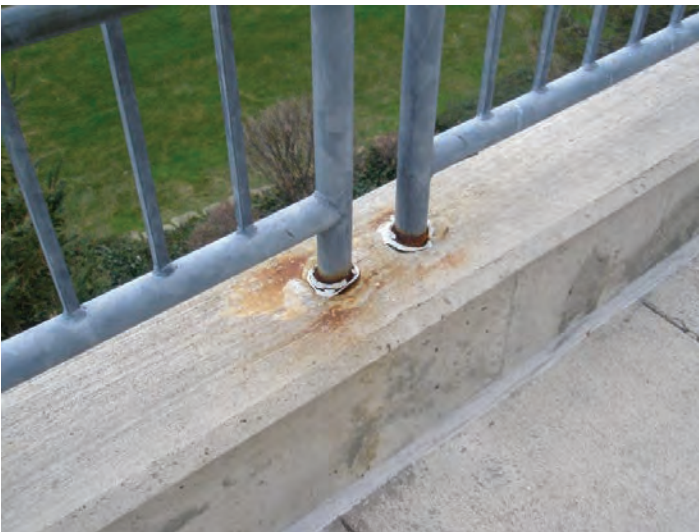
C2 - Typical failed sealant at guardrail post
