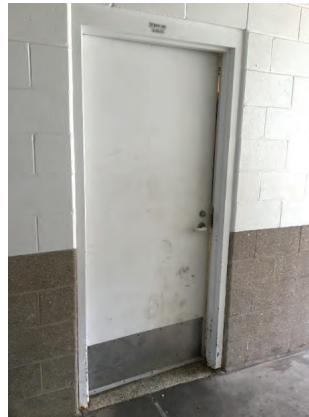
A3 - Typical hollow metal door assembly
