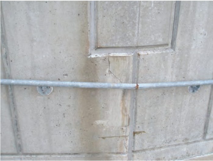
C1 - Typical Structural crack in retaining wall
