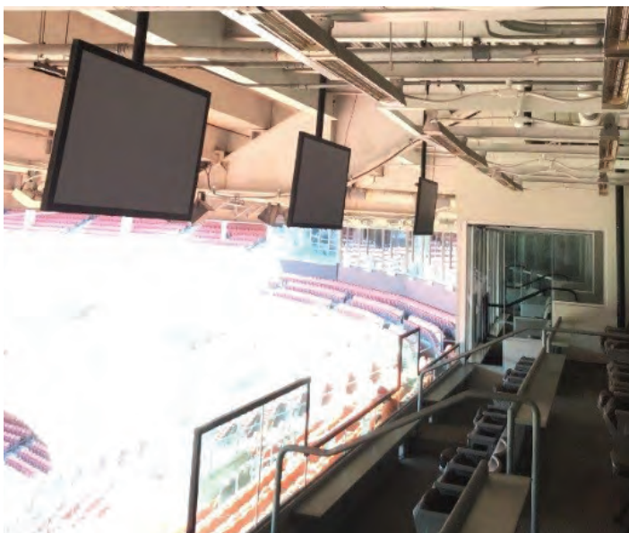
M3 - Typical Radiant Heater Layout
