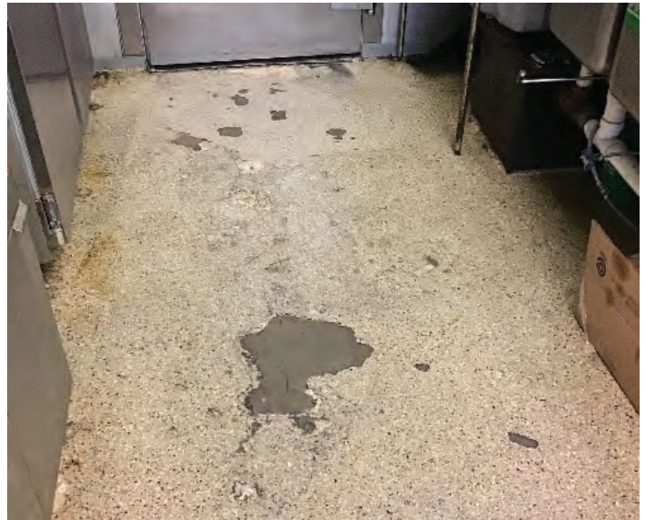
A11 - Epoxy floor in kitchen area
