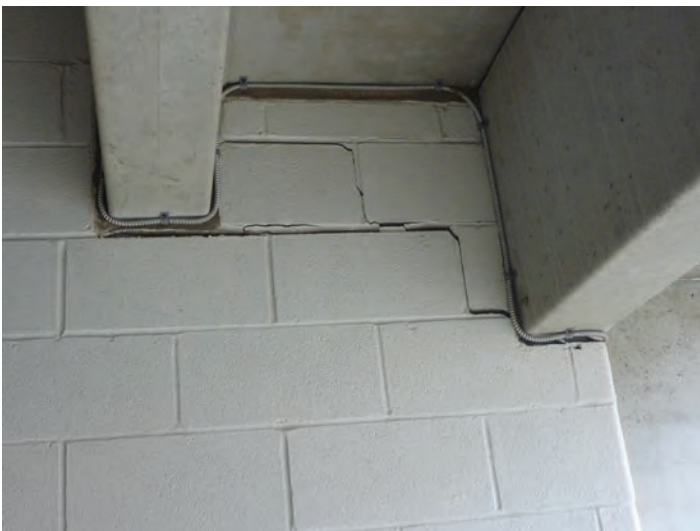
S5 - Typical Masonry Cracking at Vomitory Wall
