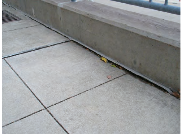
C3 - Typical failed sealant on plaza
