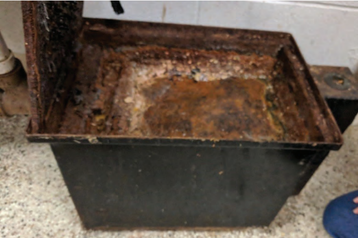
P6 - Rotted Grease Trap
