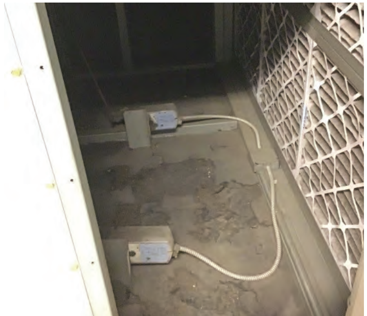
M2 - AHU Deteriorating Internal Lining
