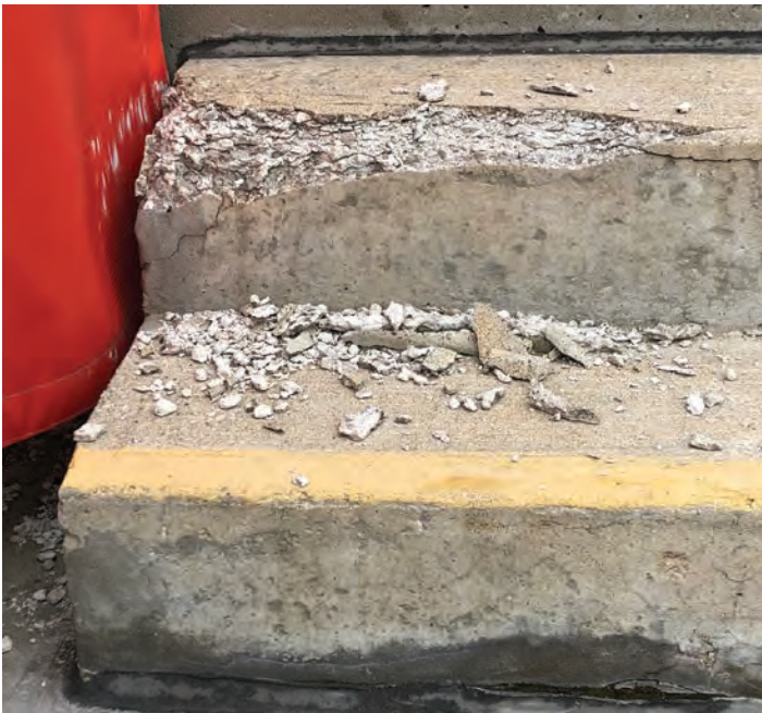
S4 - Typical Deteriorated Aisle Step
