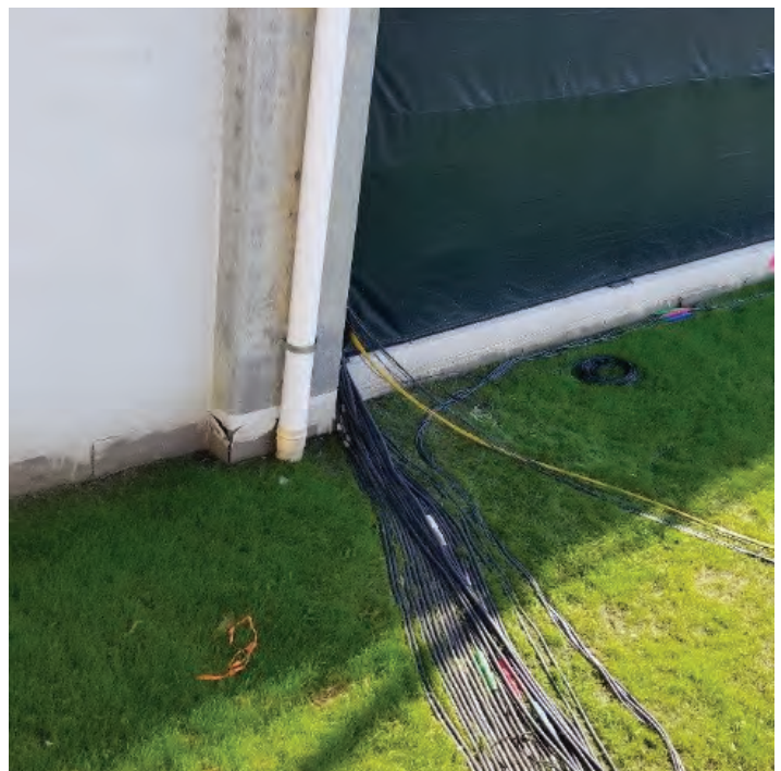
E16 - Temporary power cables entering service area
