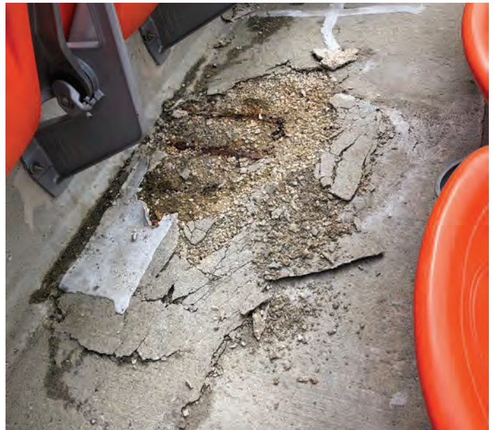
S1 - Typical Spalled Concrete
