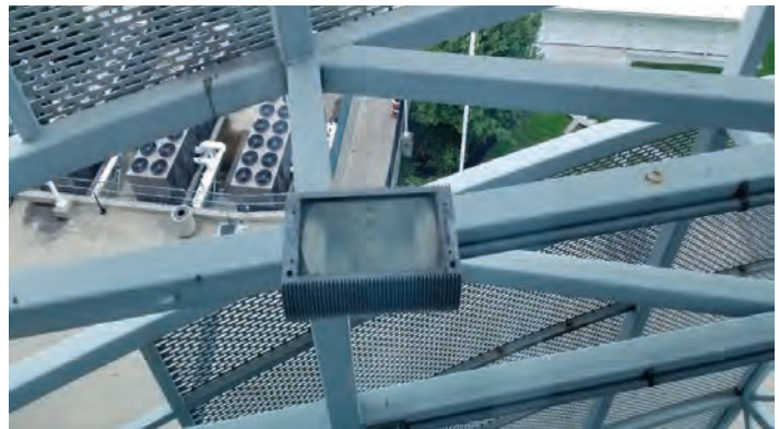
E10 - HID fixture mounted behind windscreen
