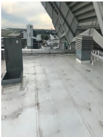
A1 - Typical single-ply membrane roof
