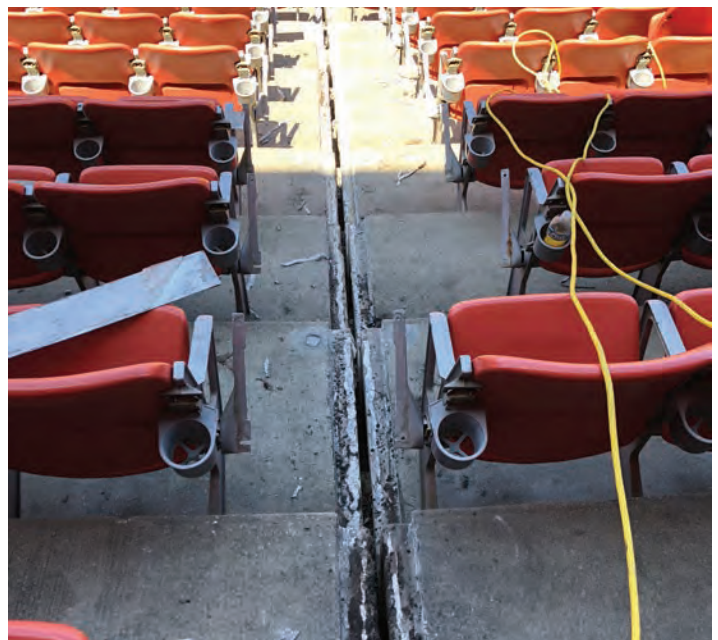
S7 - Typical Precast Joint
