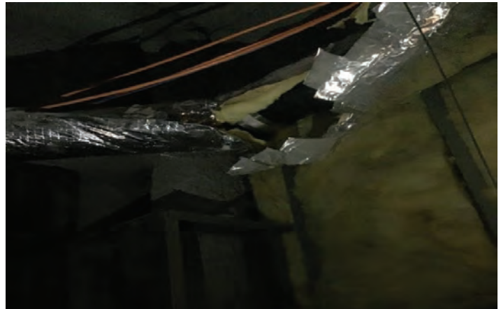
p2 - Unsecured Insulation in Suite Level Ceilings
